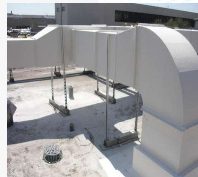
Duct cladding
